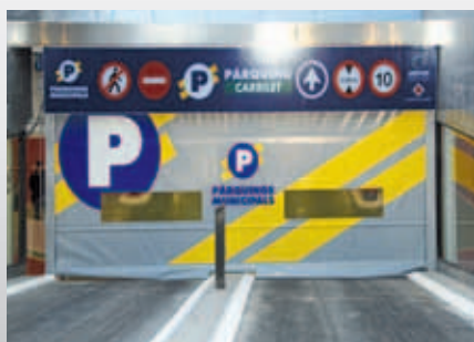
High speed door for parking access.
