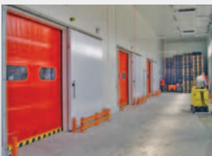
High speed door combined with chamber sliding door.
