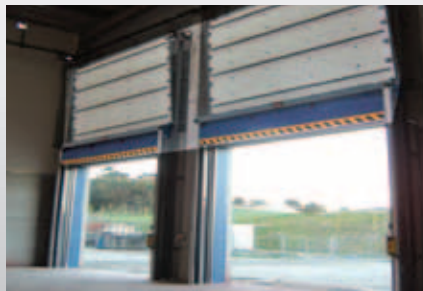
High speed door combined with sectional door.
